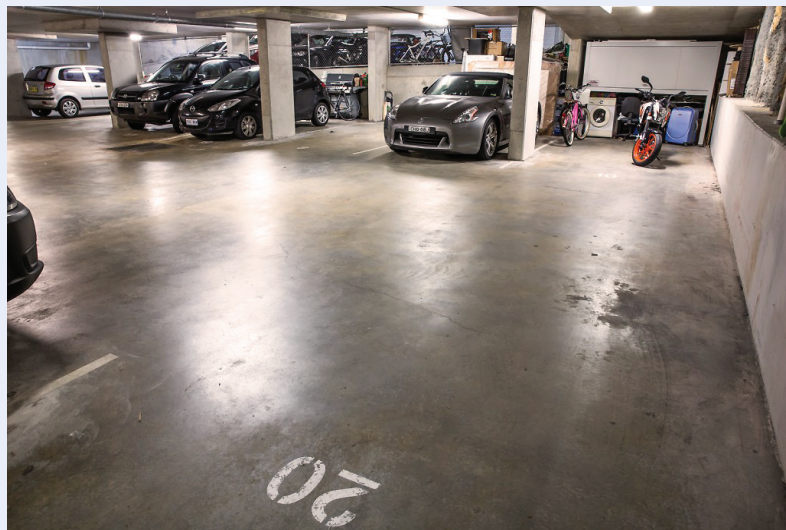
Паркінг Pittwater Road Residential Manly, Australia
