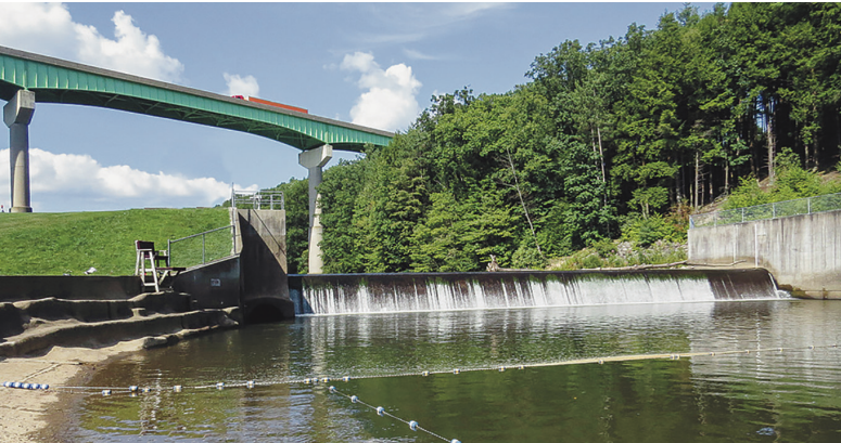
Brookville Water Treatment Plant, Brookville, PA, USA
